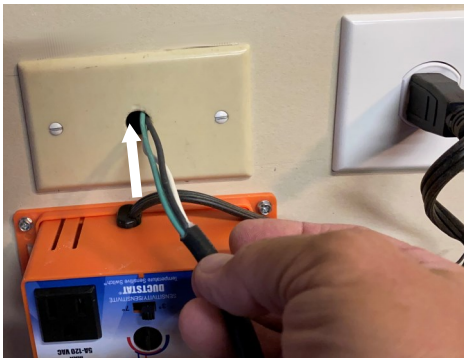
Insert garage fan outlet cord through junction box
