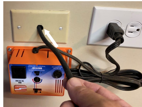
Continue to feed cord through junction box
