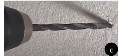
Drill marked fastener locations
